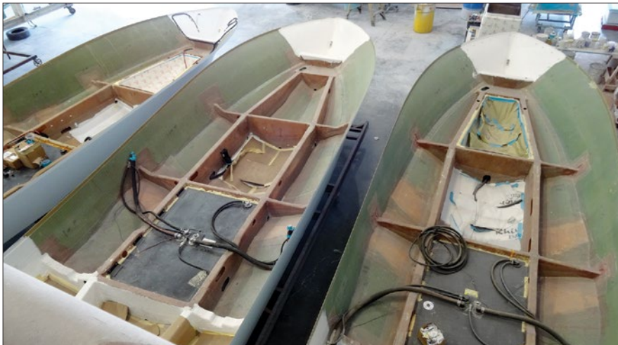
Ninety-gallon (341-l) aluminum fuel tanks are mechanically fastened to the structural grid of stringers and transverse frames before being foamed in.
